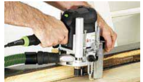
Complete removal of adhesive and seal residues when replacing existing panes with double glazing.
